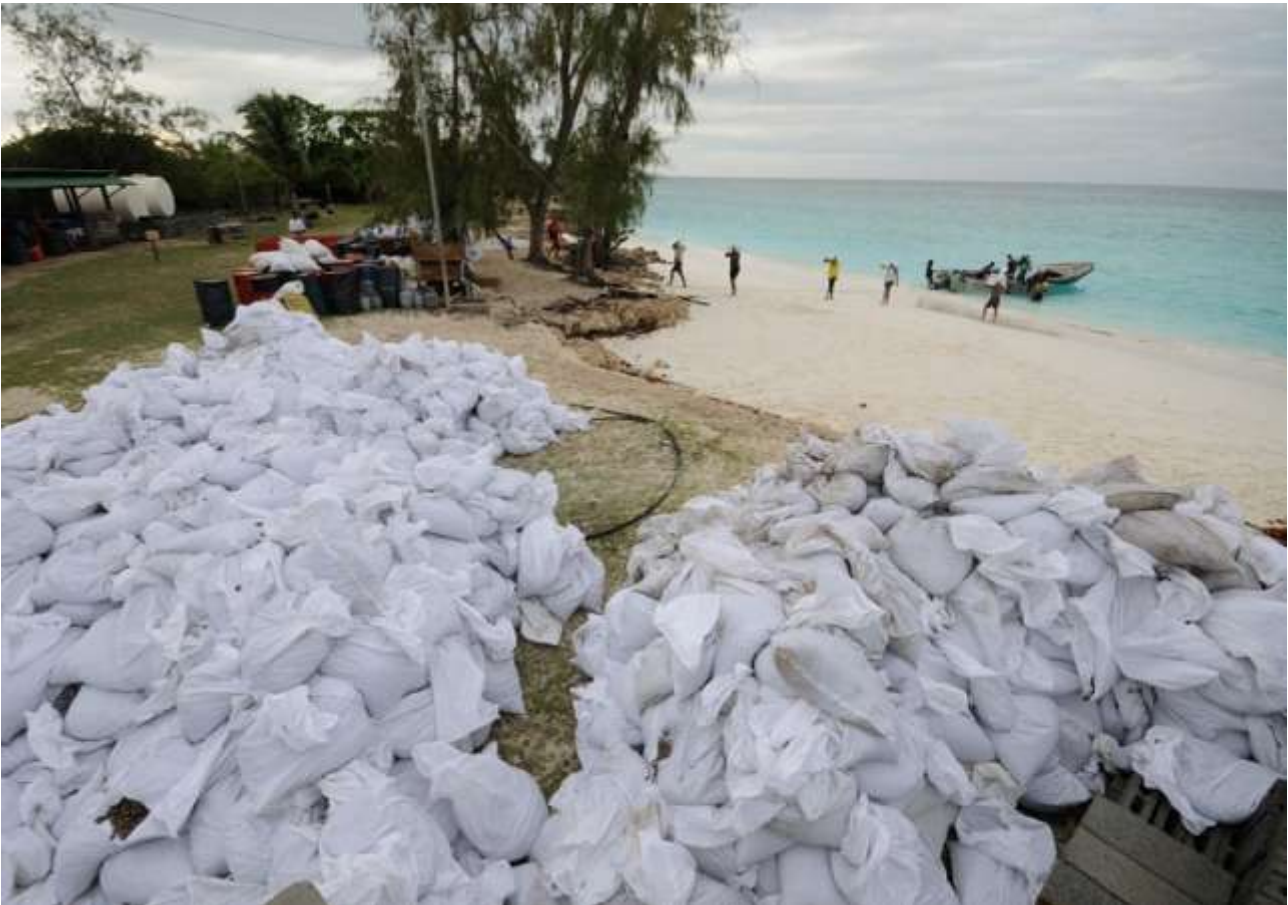
Unloading of construction materials on Aldabra © Michal Sur (December 2011)
