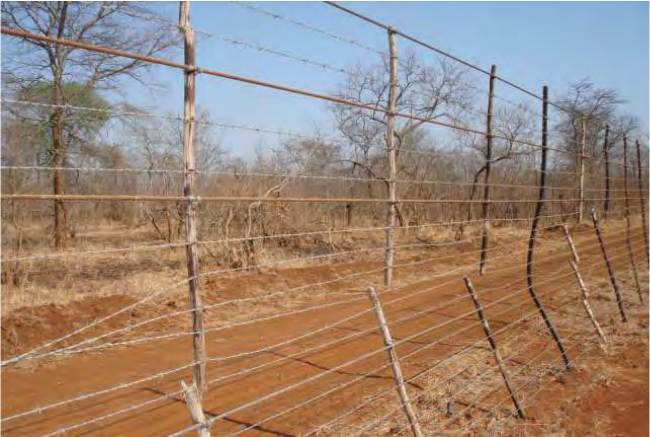
New fencing damaged by elephants at Kruger National Park © Ken Ferguson
