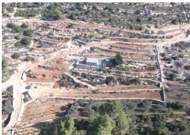
Figure 2. Drone image of a destructive local practice in a rich biodiversity area in which bulldozers imported stone and soil to construct poorly engineered terraces and roads that blocked the natural flow of water in the valley.
