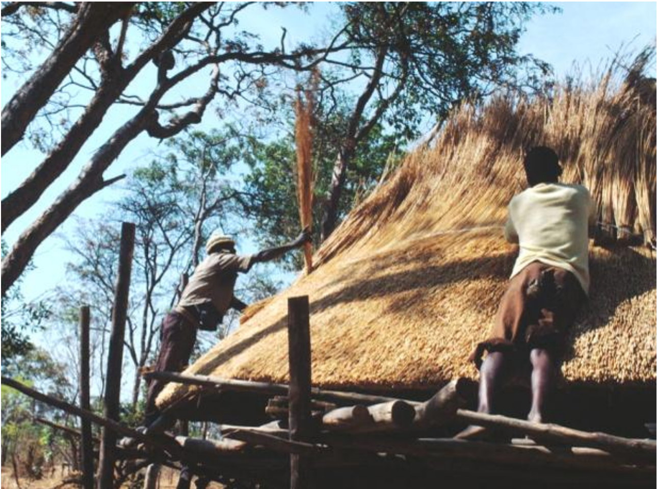
Traditional thatch being put on education facilities building in Kasungu National Park, Malawi © John E. Newby / WWF-Canon
