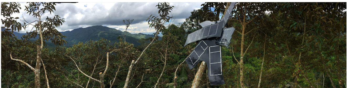
Solar panel and acoustic sensor mounted in the canopy © James Reed
