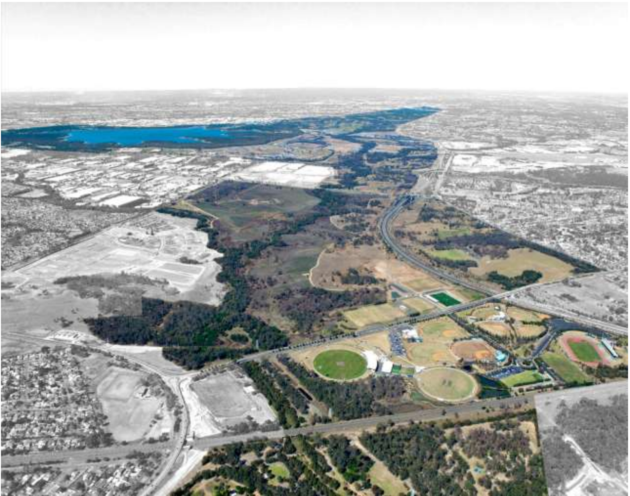
Figure 2: View south over northern portion of Parklands
